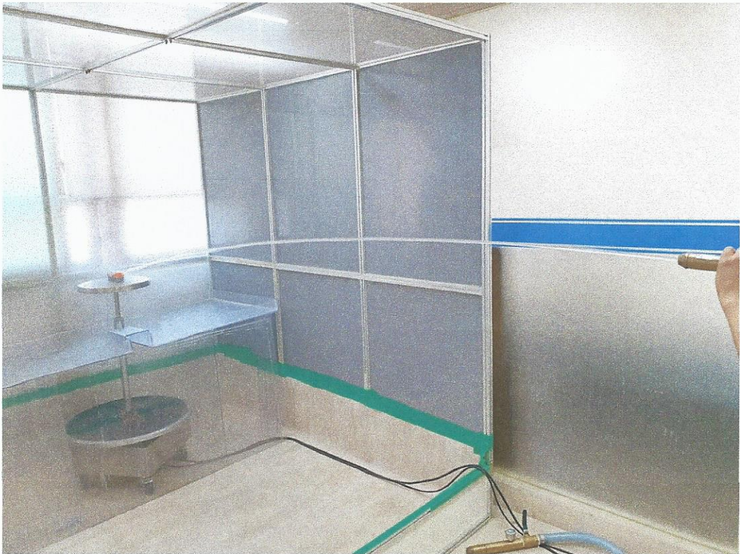
[Photo 5 - during the waterproof test]
