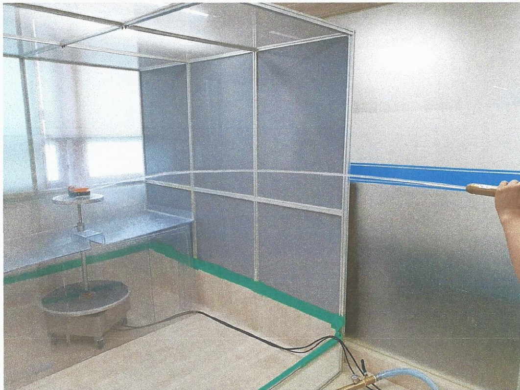
[Photo 5 - during the waterproof test]
